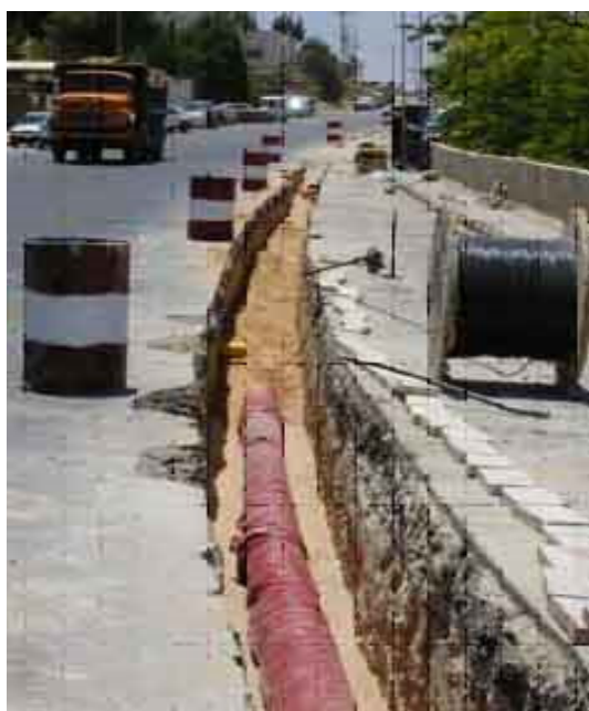
Rehabilitation of Amman Water Network Project – 2003 (partially funded by USAID)
