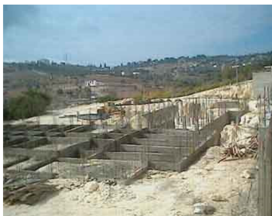
Construction of a School in Tafieleh Governorate/ ERfKE
